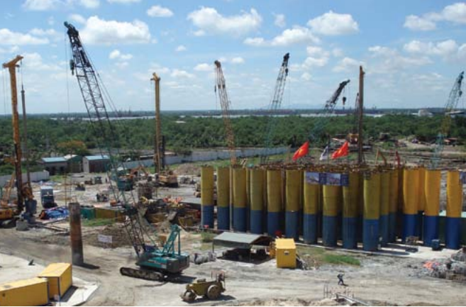
EverRich Apartments, Ho Chi Minh City, Vietnam
